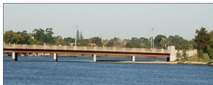
Perth Causeway Bridge
