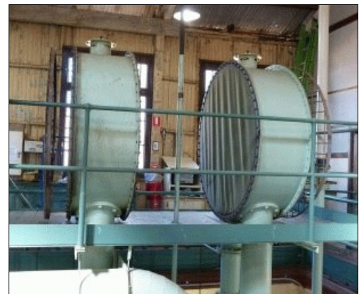
Producer gas charge holders at Cobdogla
