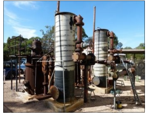
Producer Gas Plant at Cobdogla Steam & Irrigation Museum
