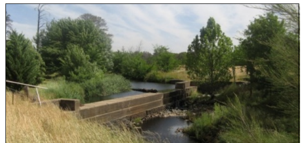
Canberra Main Outfall Sewer crosses Yarralumla Creek. Image - EA
