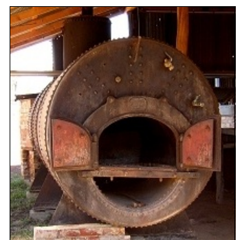
One of the disused boilers still at the woolscour.
