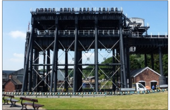
Side view of the Anderton Boat lift.
