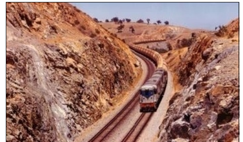
Wheat train on the dual gauge track passing through a cutting in the Avon Valley Image - EA
