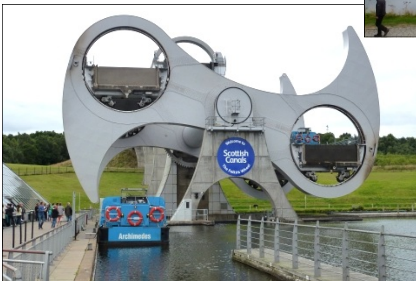
The Falkirk Wheel in mid-rotation, viewed from the North near the Union Canal entrance, showing the end of a canal boat lined up to enter the caisson. Photo Keith Baker
