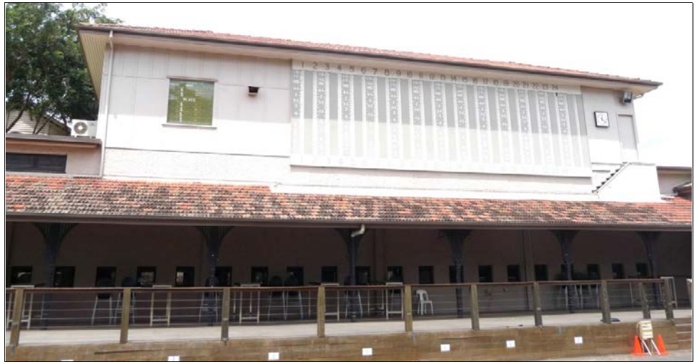
The New Farm Tote building in 2012
