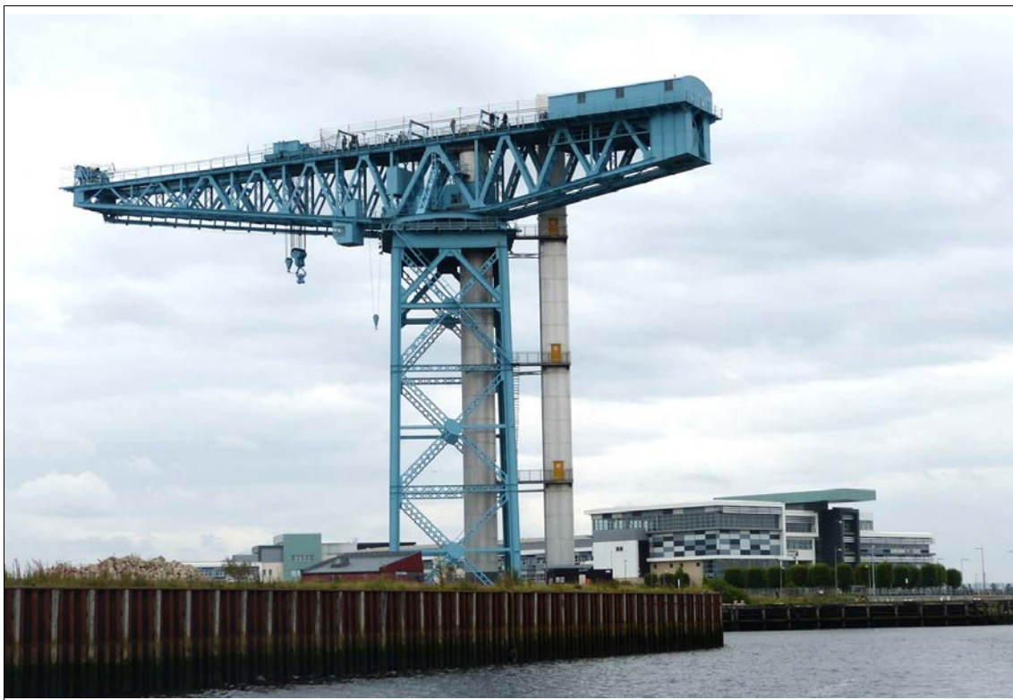
The Clydebank Titan Crane viewed from the water. The shafts for the stairs and lift built for the bungy jumping operation can be seen behind the tower. The visitor centre is the grey-roofed red building at the base of the tower. New college buildings are in the background. Photo Keith Baker
